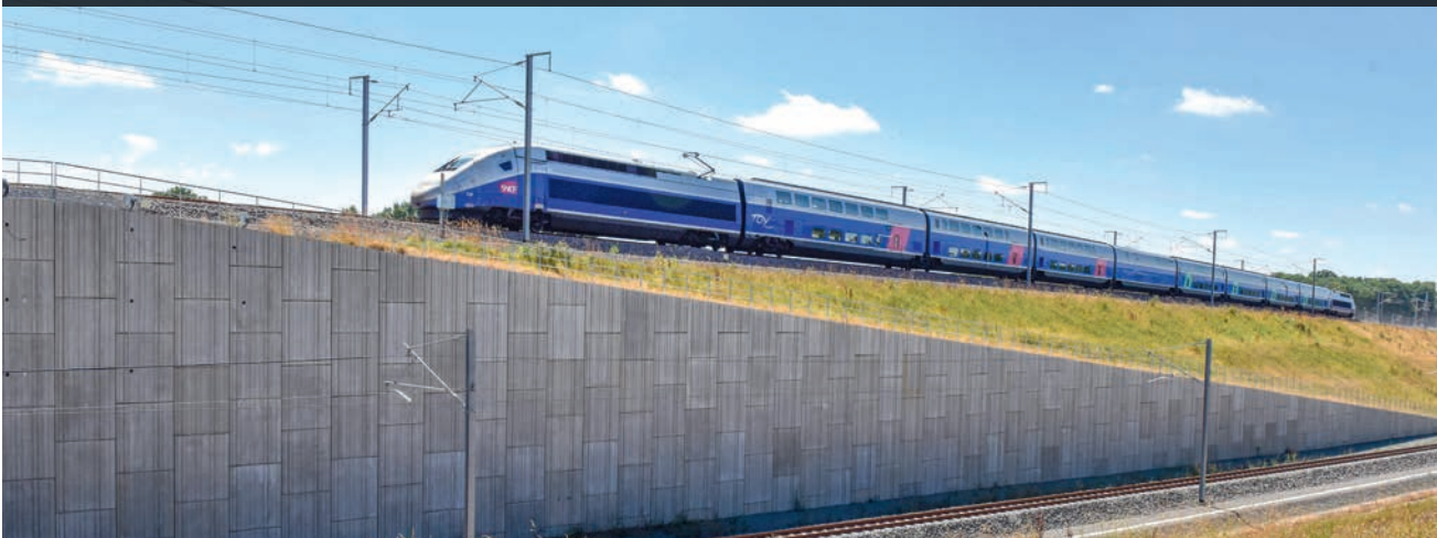
Reinforced Earth® walls along the Paris-Bordeaux high-speed rail line, France
