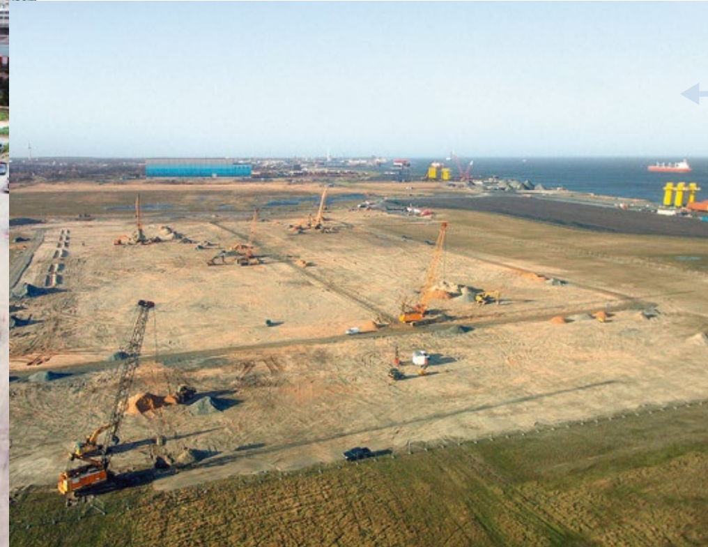
The Australian teams implemented 58 jet grouting columns
