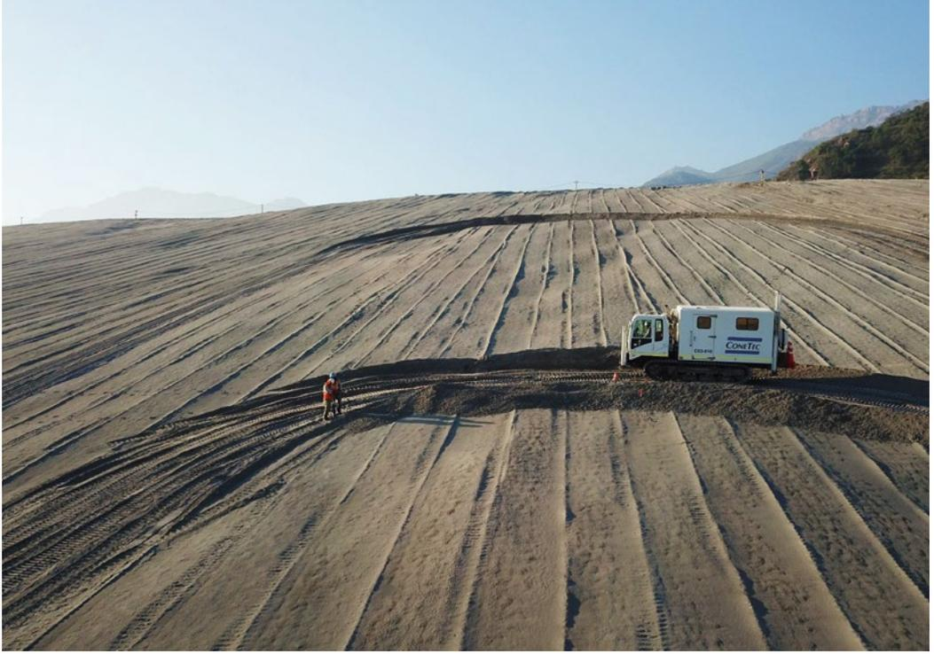
The teams at ConeTec carried out a geotechnical site investigation of a large mine tailings dam in Chile. They carried out seismic piezocone penetration testing (SCPTu) and installed push-in VW piezometers to depths of up to 100 metres. The primary purpose of the investigation is to monitor the stability of the dam. The goal was to safely provide high quality geotechnical information to support engineering decisions.
