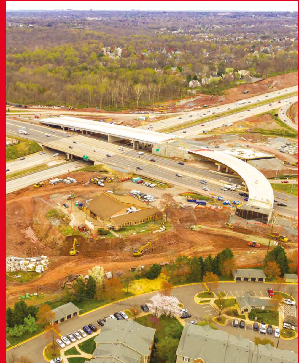
© Work was performed as a subcontractor for FAM Construction on the Transform 66 Outside the Beltway project
