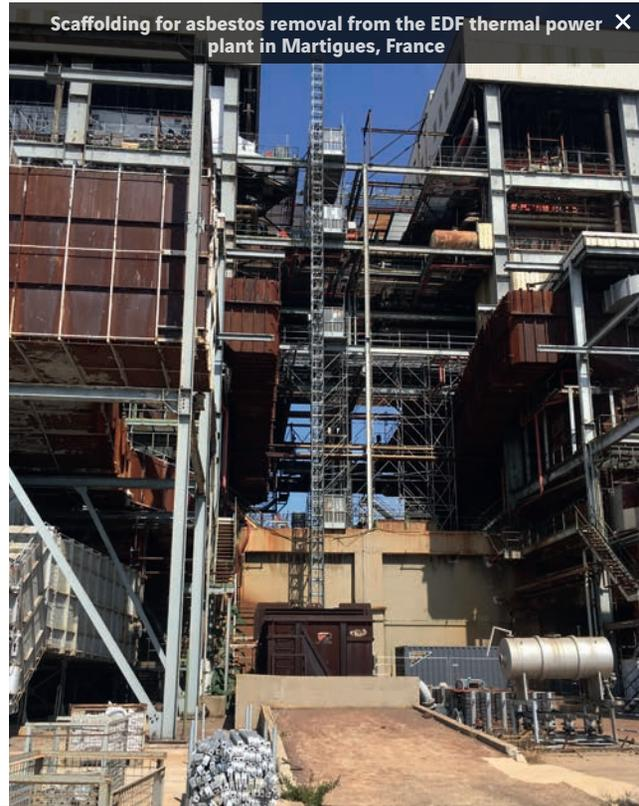
Scaffolding for asbestos removal from the EDF thermal power plant in Martigues, France
